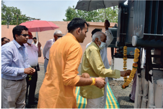
Inauguration of Electric Subcentre
